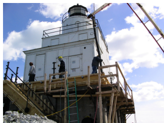
Lighthouse Renovation Manitowoc, WI
