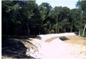
Oscar Street Easement Storm Sewer and Drainage Ditch
